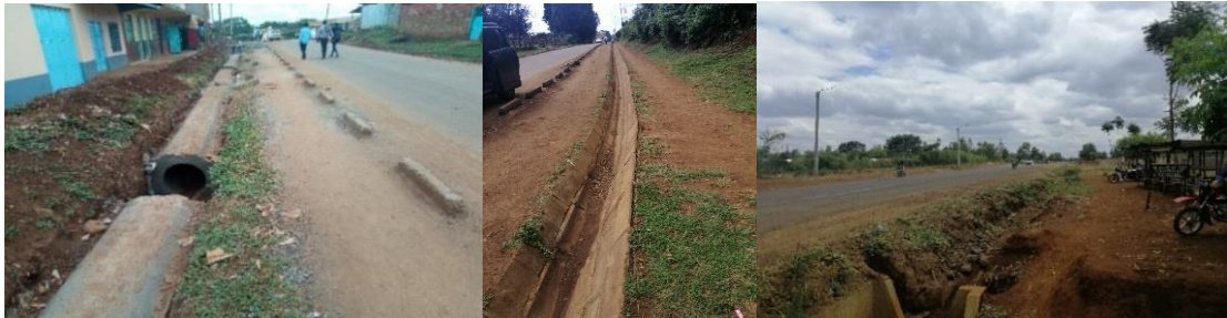
Plate 6-10: Closed drains in Kutus, open concrete and earth drains in Kerugoya Town
