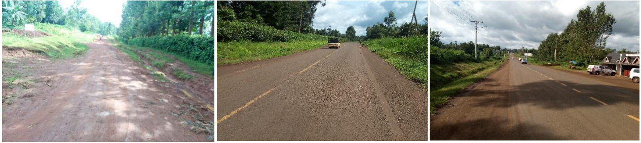
Access road in Ithare, Rukenya-Kabare Road, Kutus, Kerugoya (B27) road.
