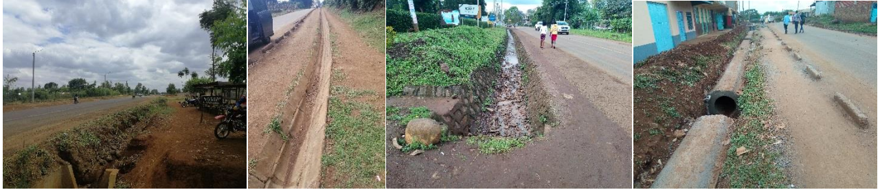
Open storm water drains (earth and concrete) in Kerugoya and a closed storm water drainage in Kutus
