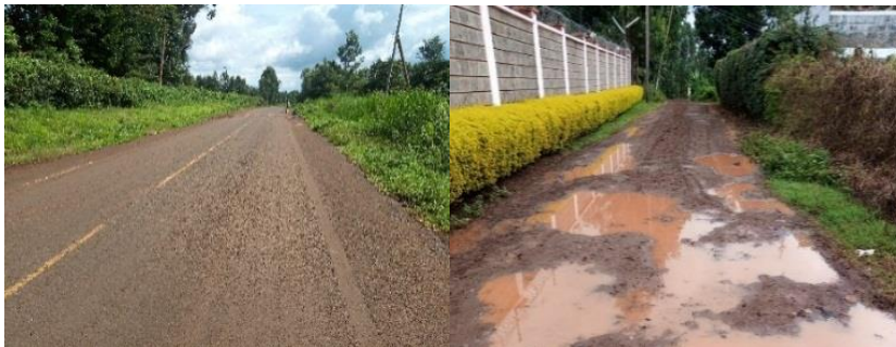
Plate 8-1: Rukenya-Ithare Road and an access road in Kerugoya
