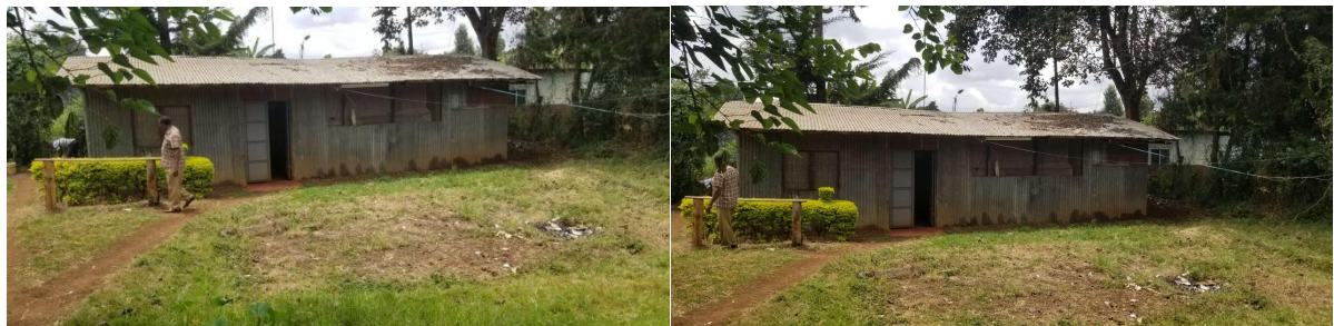
Fig 2. The current Fire Station Headquarters
