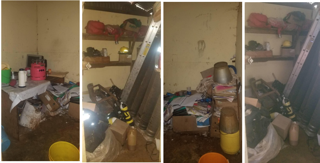
Fig 5. The current Fire Station storage area. The Kitchen also serves as a storage area.
